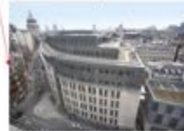
St Bartholomew's Hospital, London, Opened in June 2016
