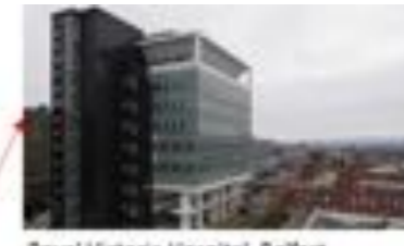
Royal Victoria Hospital, Belfast Phase 2b 2015
