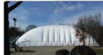
G POOL AIR DOME SWIMMING
