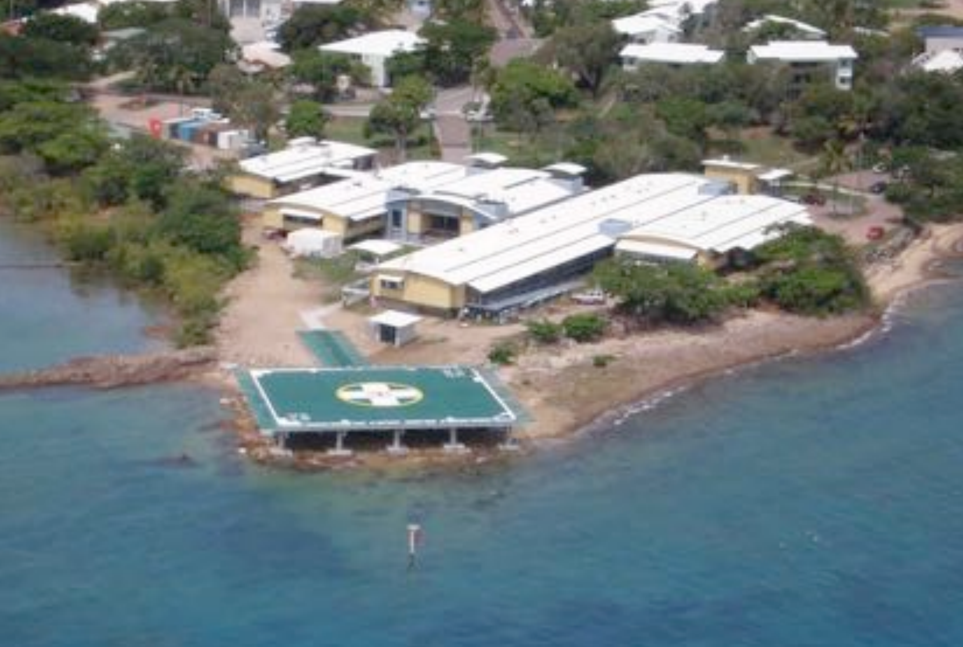
Thursday Island – New Helipad completed December 2010
