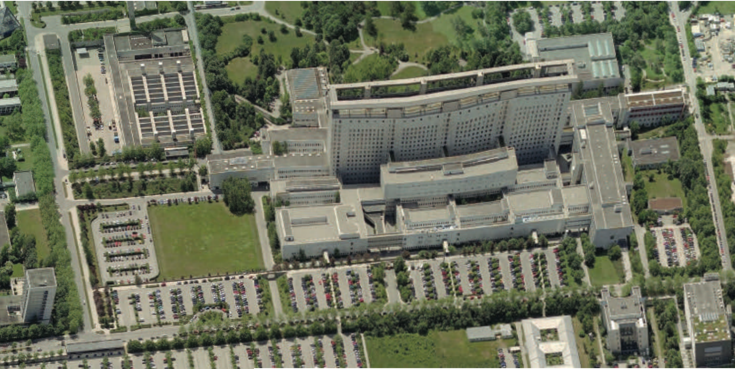
University Hospital Grosshadern, Munich: built 1967-77
